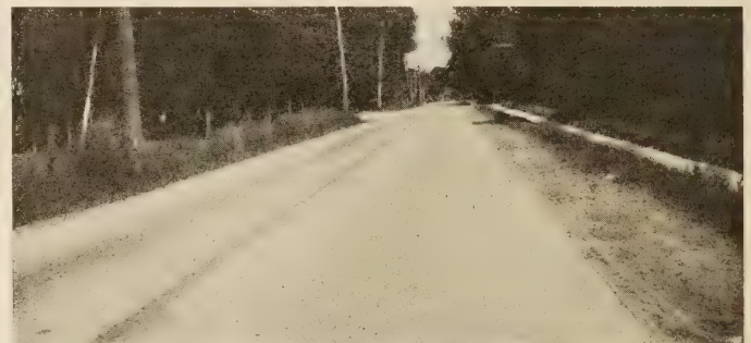
FIG. 16.—Test 1, also on an 18-foot concrete road, shows the loss of effective width caused by the low shoulders. Compare with roads of the same width but good shoulders shown in Figures 5, 17, and 18
